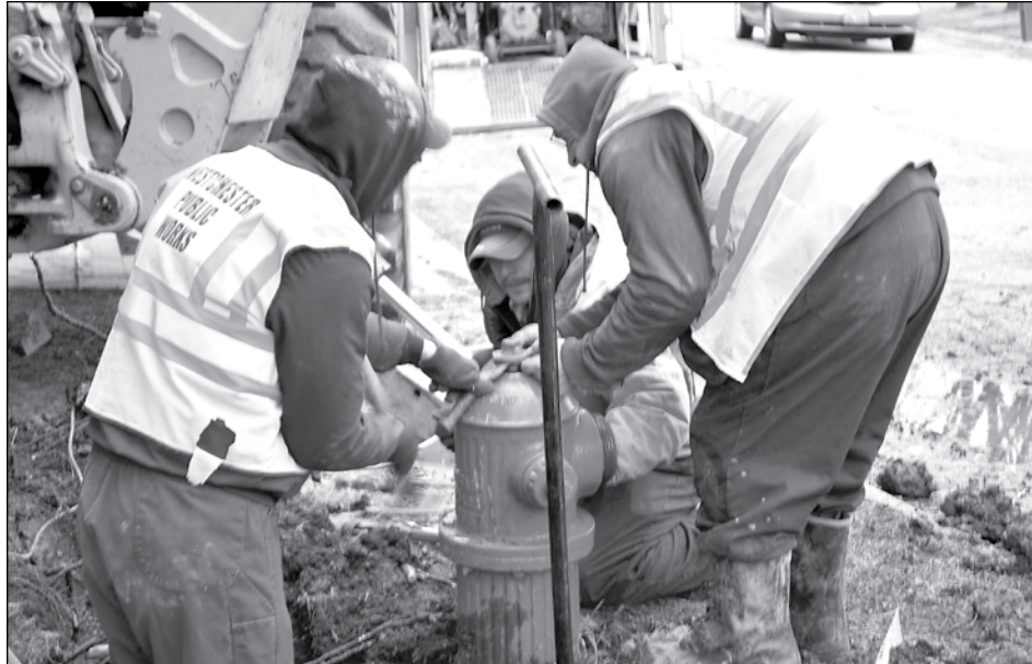
Public Works employees diligently repairing a valve.
