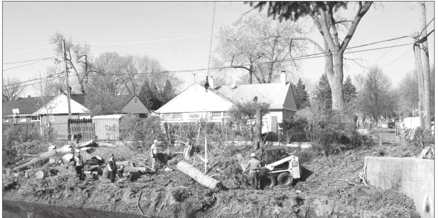
Public Works and Sinnott Tree Service, Inc clearing Addison Creek
