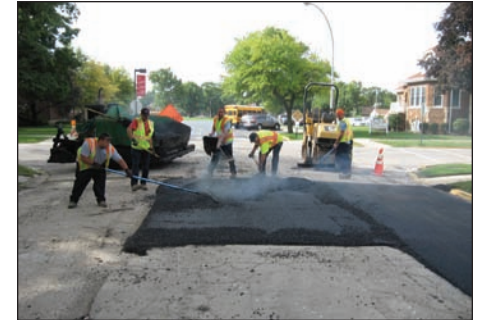
Public Works crew paving the streets of Westchester.
