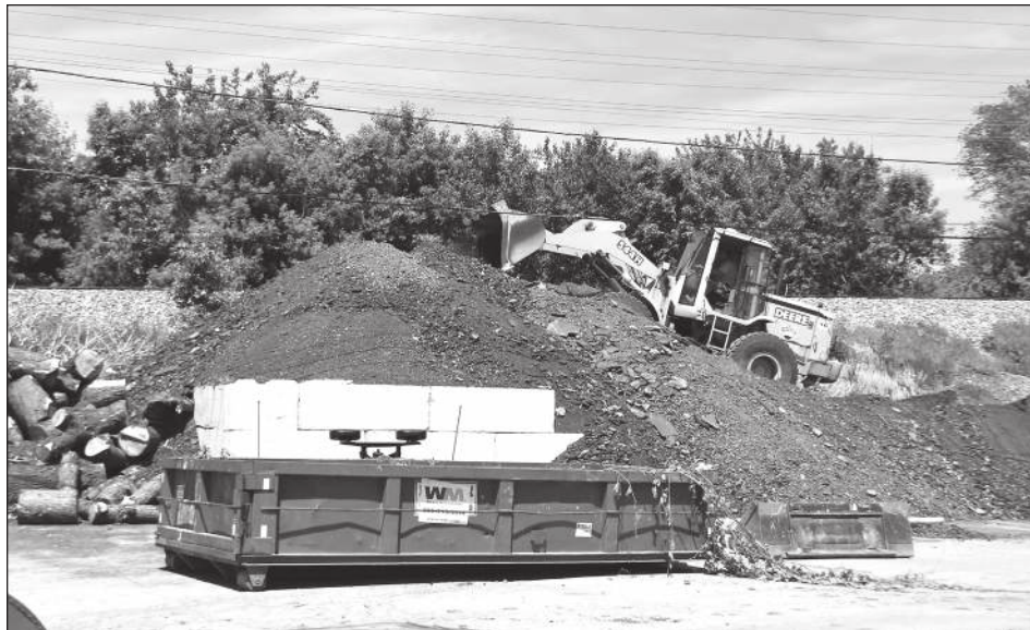
Asphalt grindings being stockpiled for reuse in alleys or as fill.
