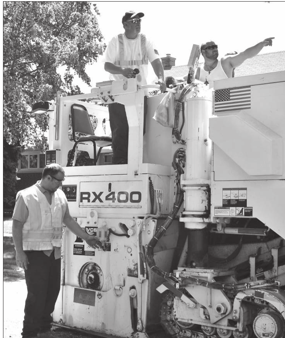
Westchester public works crew operating the grinding machinery.
